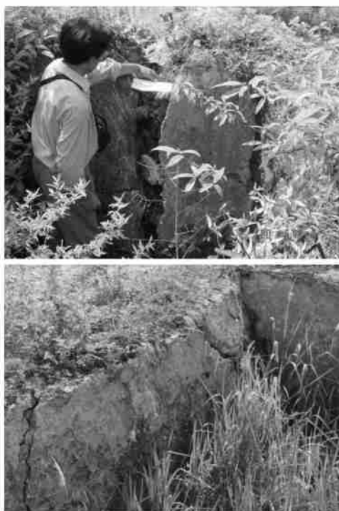
照片5 水池边缘开裂,裂缝最宽处超过20cm Photo 5 The crannies in the brinks of the pool, the widest cranny is wider than 20cm
