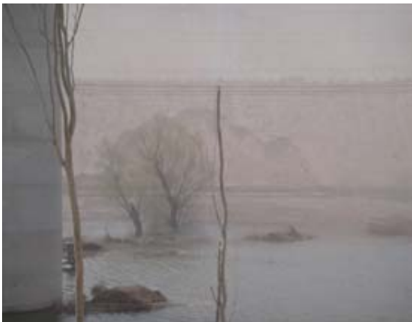
Fig.1 Engineering site photos
