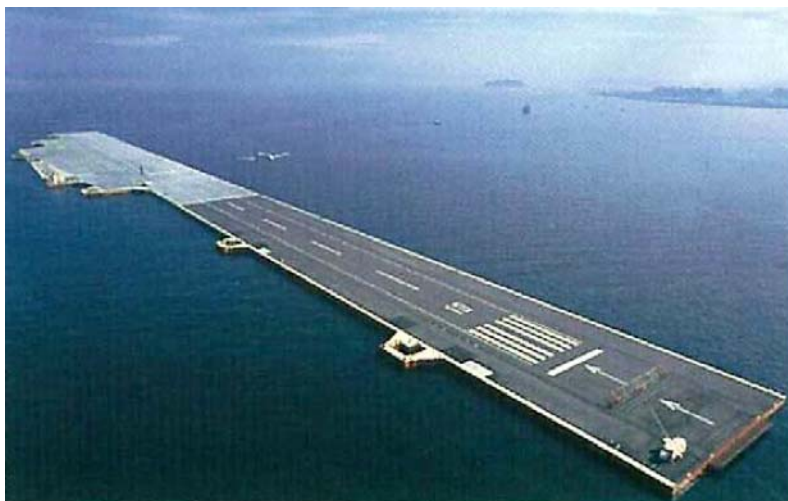
图一: Mega-Float in Tokyo Bay, Japan (photo courtesy of SRCJ)
