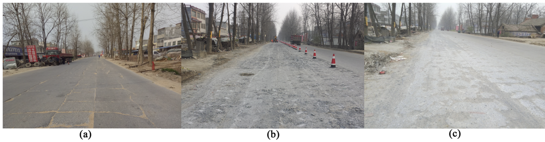
FIG. 15. Cement concrete pavement before and after crushing. (a) Pavement before crushing. (b) Pavement after crushing. (c) After debris cleaning.
