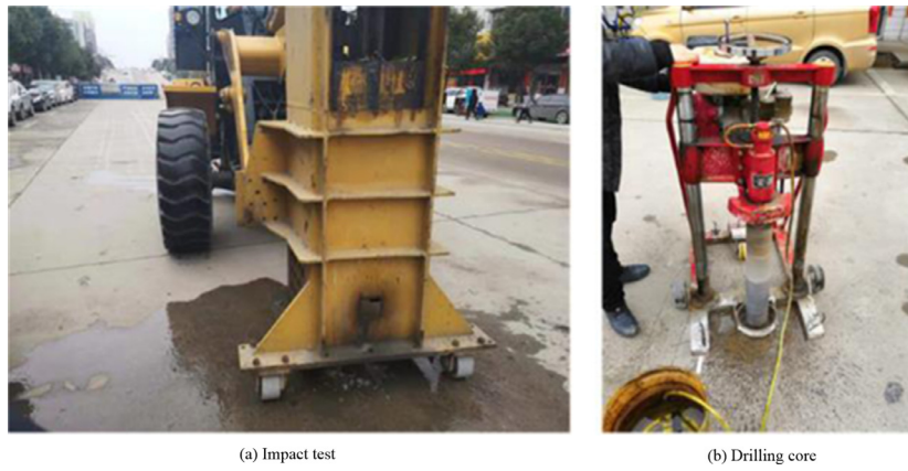
Fig. 13. In-situ impact test and core drilling of concrete pavement.
