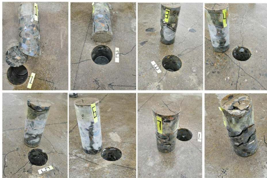
Fig. 16. Crack distributions and crack surface morphologies of the core samples.
